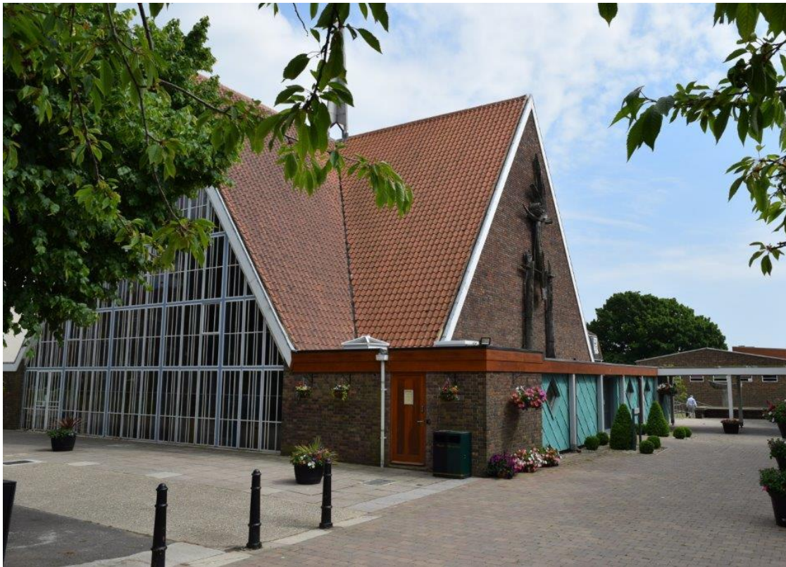
A locally Listed Building - The Chapel, University of Chichester, Bishop Otter Campus
